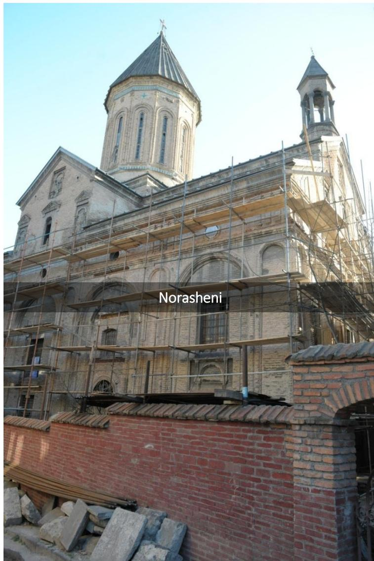
Representatives of the Georgian Diocese of the Armenian Apostolic Church said only reinforcement activities were conducted in Norasheni by now. According to official data, the following work was done in the church: steel-concrete belt was installed around the whole basement; the dome was also reinforced by the steel-concrete pillars.
