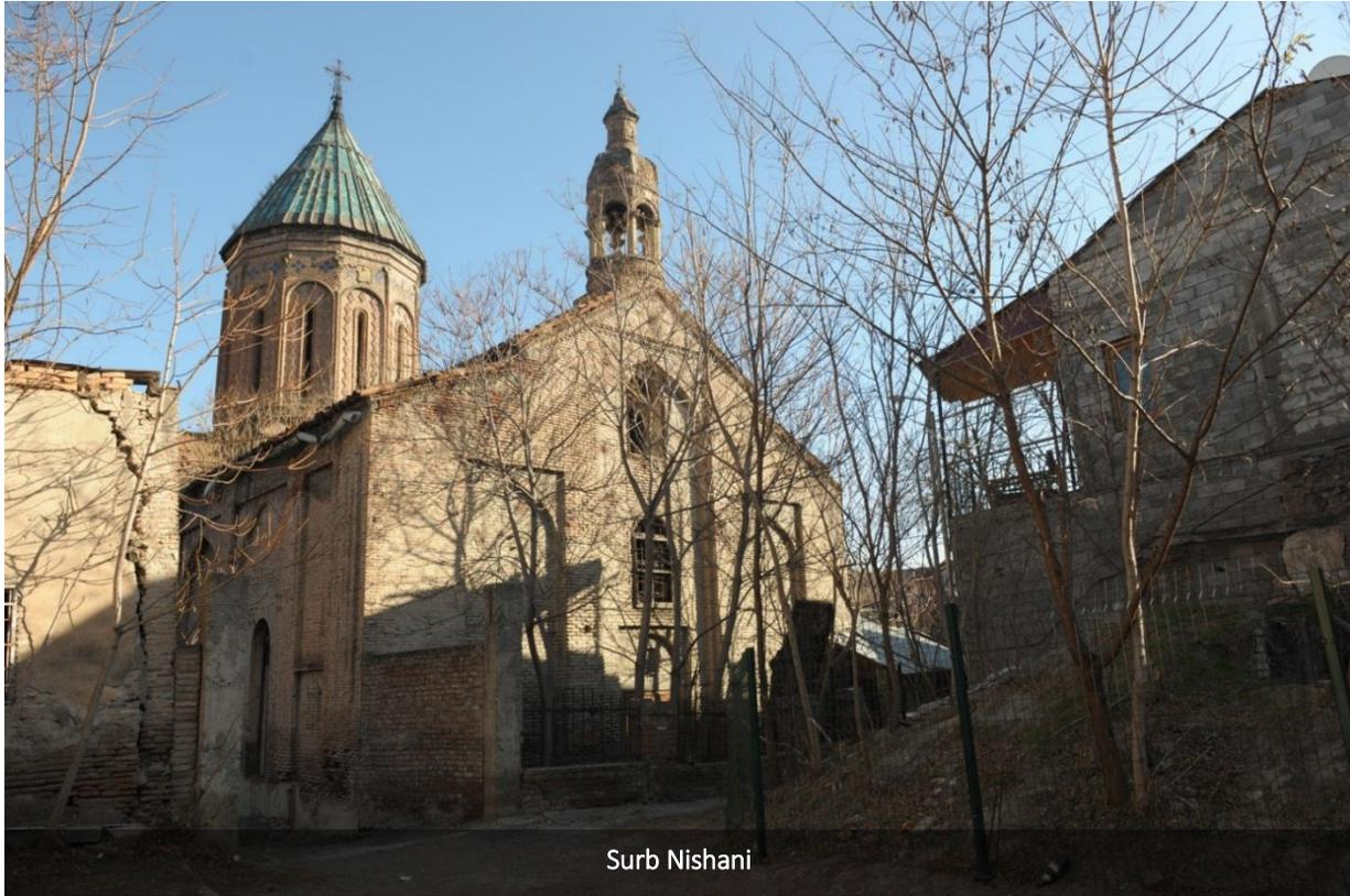
Namely, pillars and arches of the Church were reinforced by iron constructions, after what steel reinforced concrete slabs were poured into the basement. Since then the works stopped because the Tbilisi City Hall could not evict a citizen, living in the house to the south of the church.
